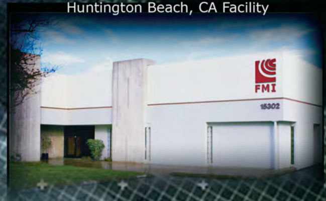
Huntington Beach, CA Facility
